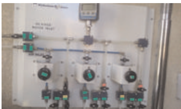
Panel de Control
